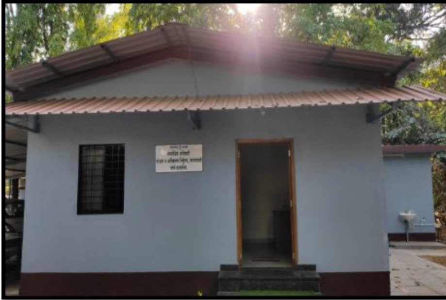
RFO Mobile squad office renovation 2024-25
